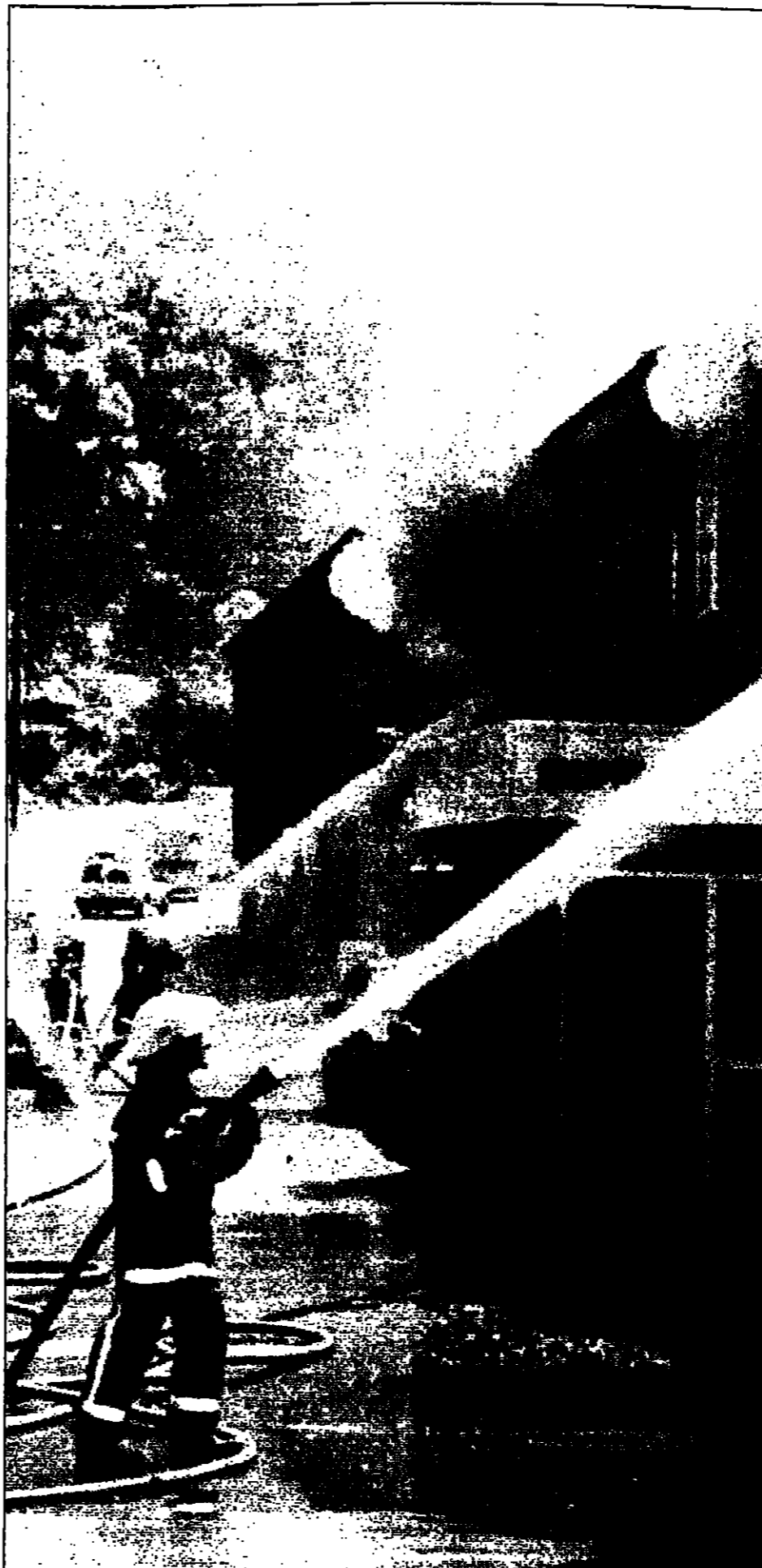
A fire at Coutant Lambda, a power supply organisation in Ilfracombe, Devon, destroyed nine offices in 12 minutes. The company was functioning the following day thanks to Granada Business Continuity which supplied equipped mobile offices
